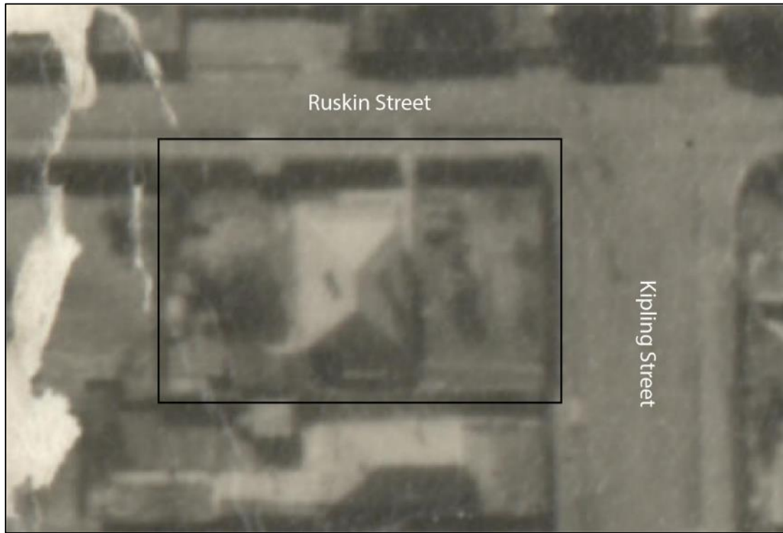
Figure 2. Aerial photograph of 30 Ruskin Street taken c.1955-1959. The approximate area of the property owned by Froggatt and Manifold is outlined in black. Image: modified from aerial imagery available on canterburymaps.govt.nz
